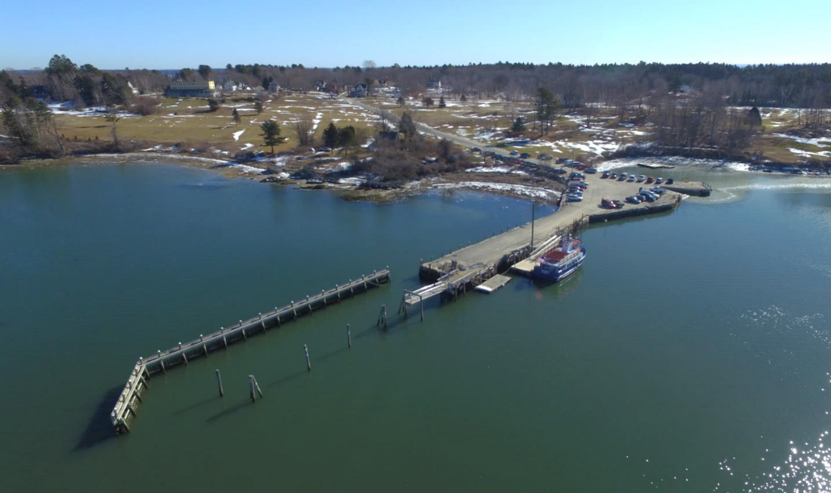
Stone Wharf from above; Picture courtesy of Rick Harbison
