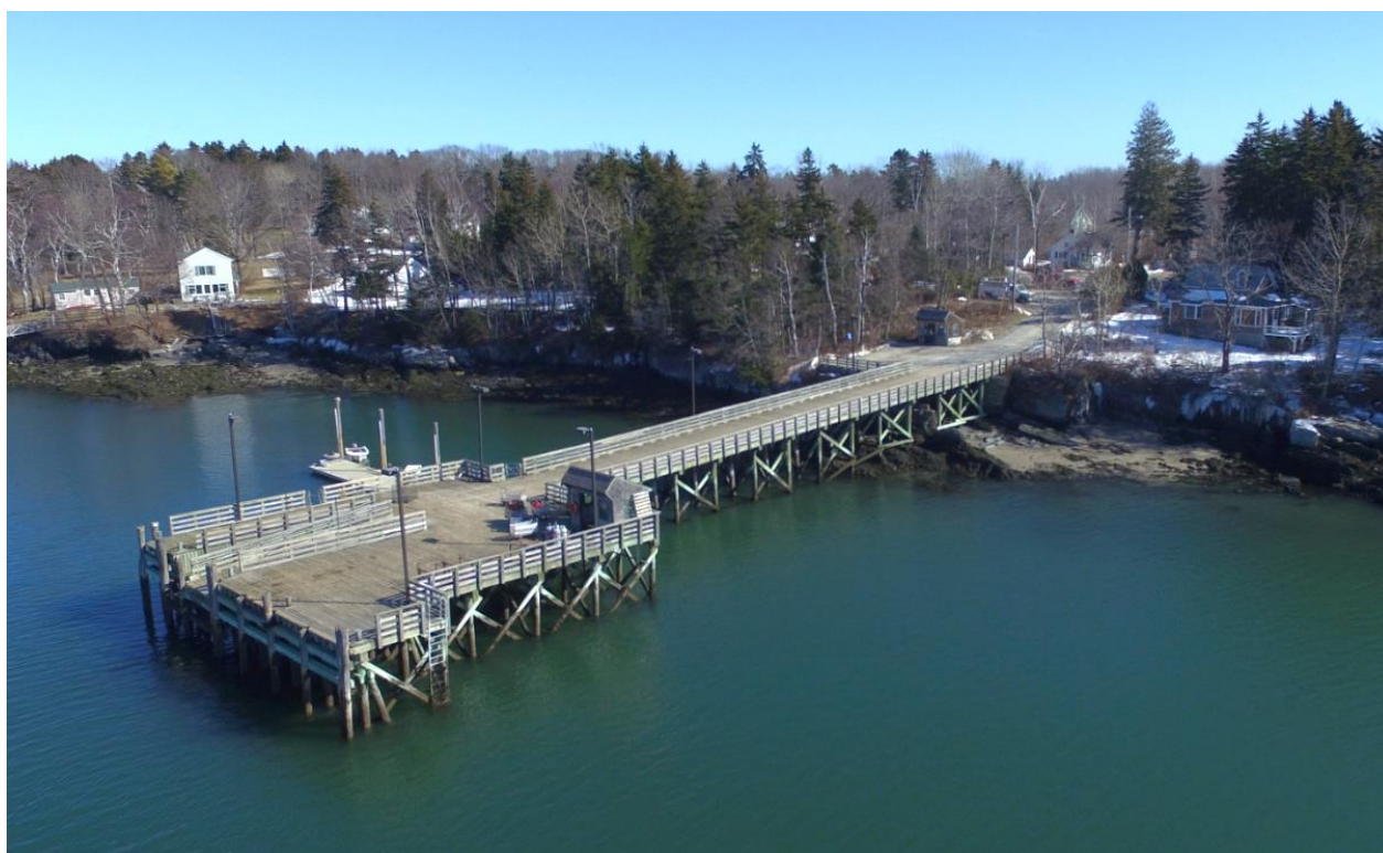
Chandler's Cove Wharf from above; Picture courtesy of Rick Harbison
