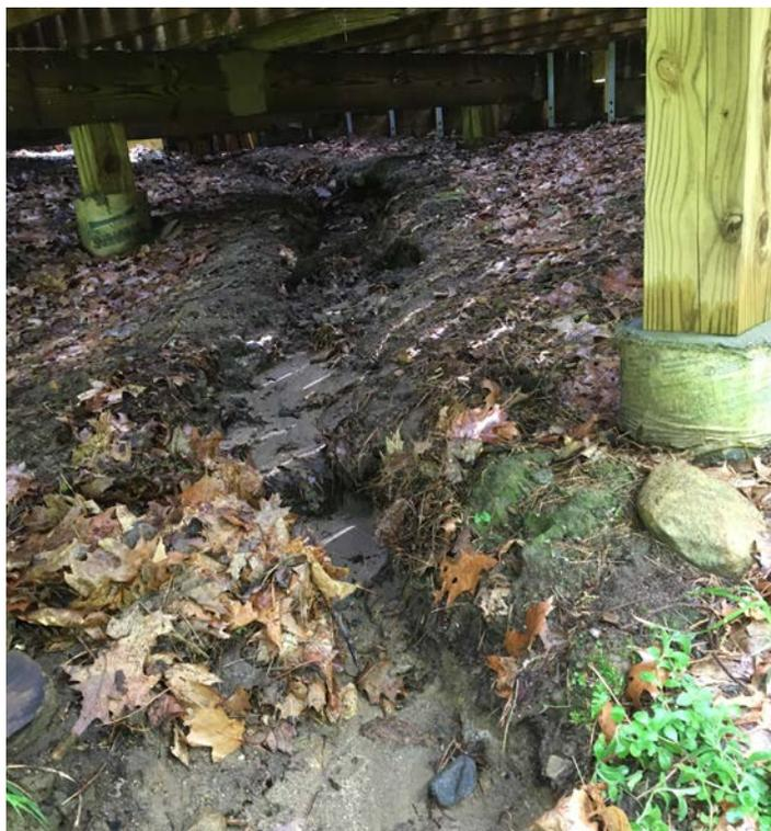
Figure 3: An example of erosion in Arrowsic (photo credit: Witham Jones)
